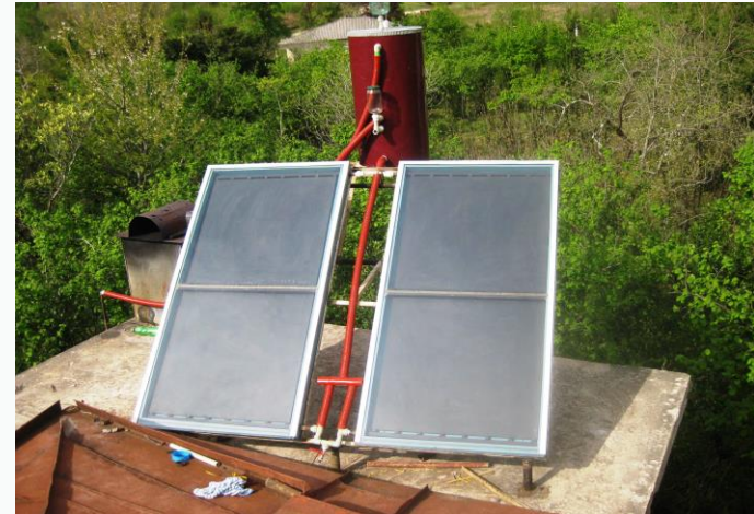
Solar Water Heaters (SWH)
