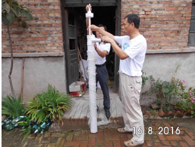
The functioning of a waste water pipe is shown by Prof. Meng at Hu village
